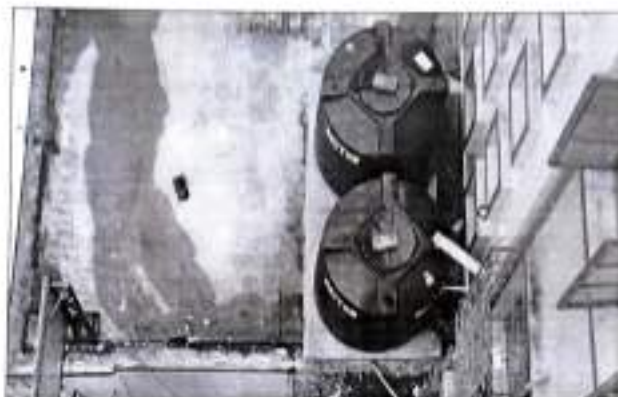
Rainwater Harvesting Tanks (1000 L each)
